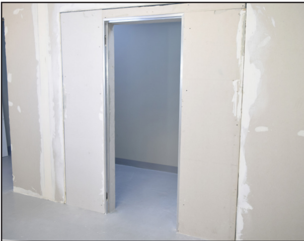
2C. Door frame with plasterboard built over it
