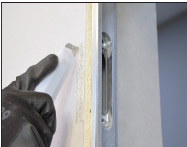
2D. In the hinge milling areas, cut the plasterboard so the hinge will fit
