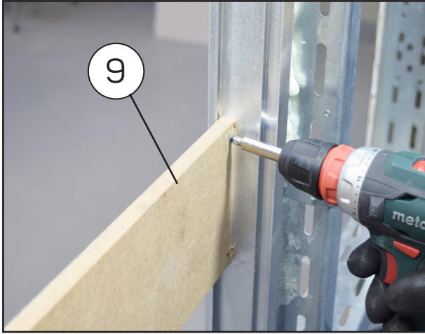
2A. Dismantle expansion strips [9]
